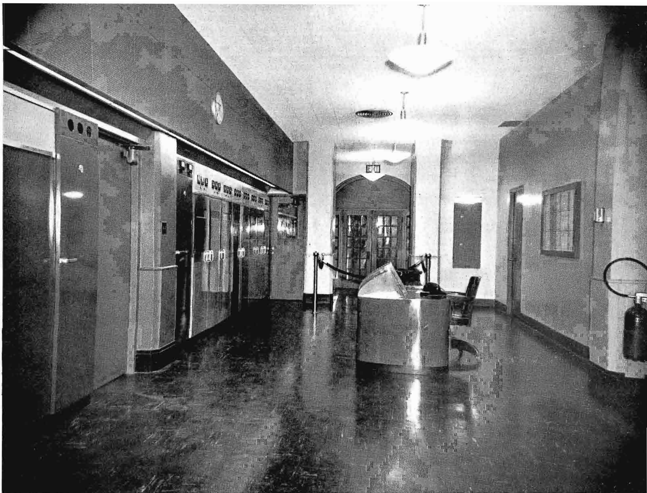
FIG. 4. The two transmitters are mounted in line as shown in this view and that of Figure 2 (which was taken from the opposite end of the room). Entrance is through the French doors at the far end.
