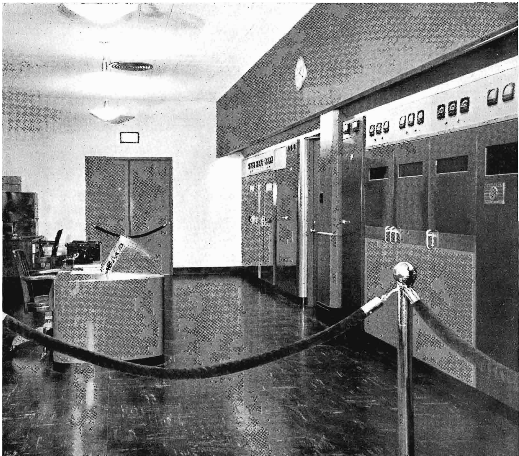
FIG. 2. The BTF-3C FM Transmitter and the TT-5A Television Transmitter are located in a first floor wing of the hotel.
