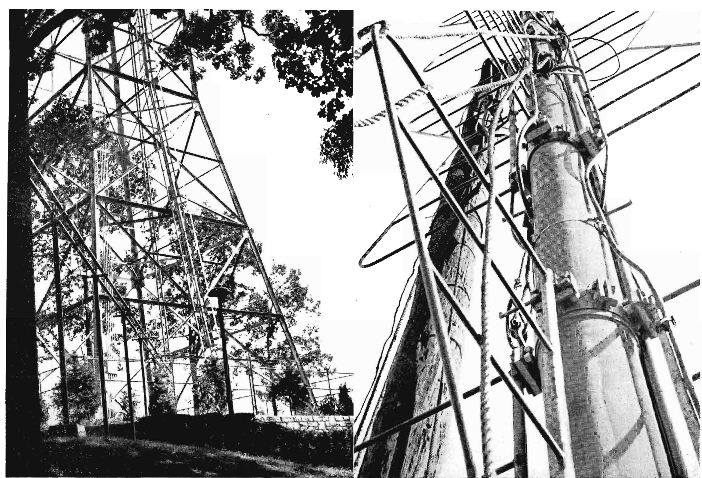
FIG. 3. The base of the antenna tower (left above) which supports the WNBW/WRC-FM antenna is less than fifty feet from the building. The view at the right above shows the 3-section superturnstile being swung into place.
