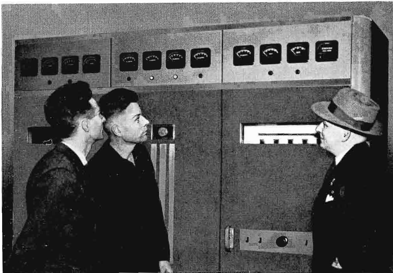
Inspecting WOPI-FM's newly installed BTB-3B Transmitter. Left to right: P. G. Walters, RCA Southeastern Regional Office; W. E. Tucker, RCA Engineer; W. A. Wilson, President and General Manager, WOPI and WOPI-FM.
