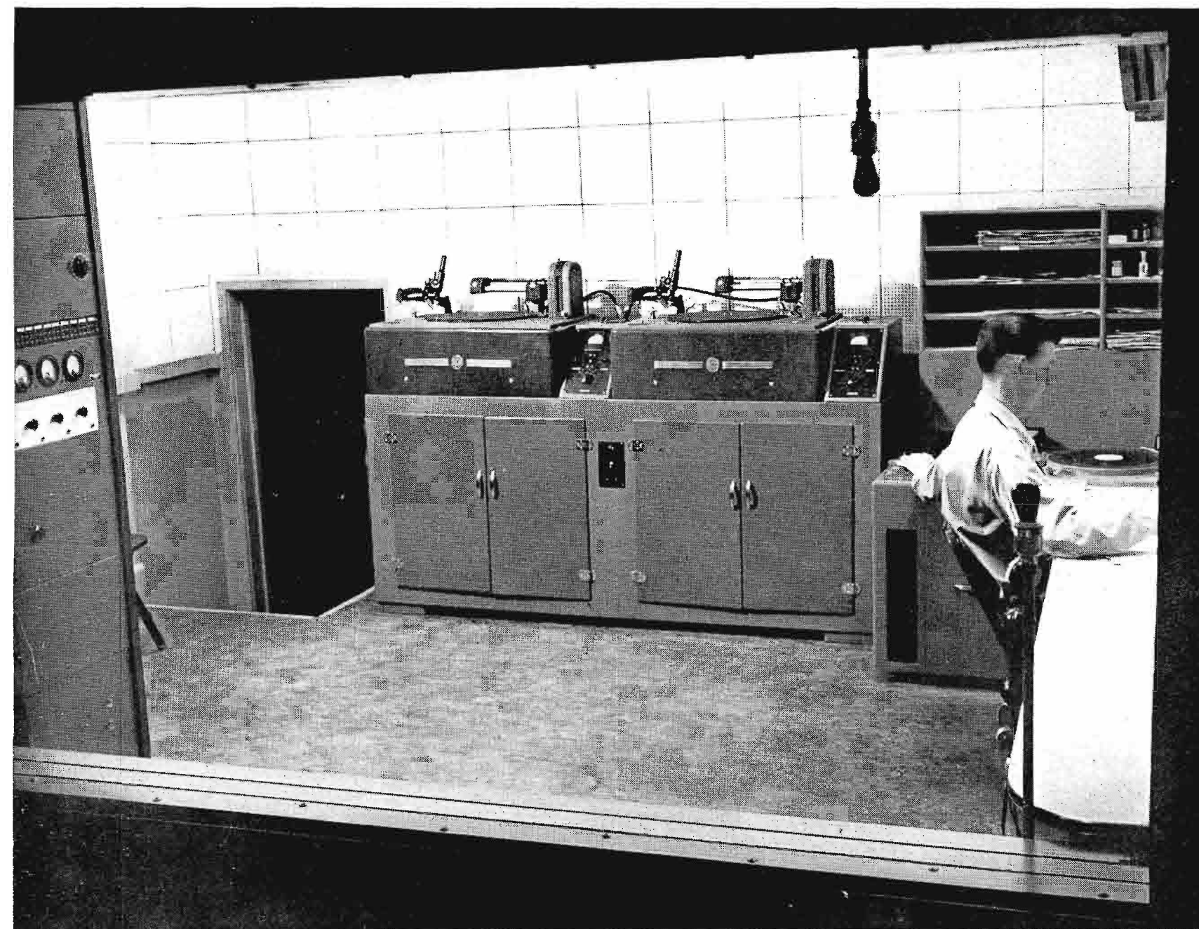
FIG. 1. RCA 73-B (Professional type) Recorders in the control room of KFBK, Sacramento, are mounted on an attractive utilitarian console which was designed and built by the McClatchy Engineering Staff. "Floating" mounting arrangement supplied with the 73-B lends itself to various types of table or cabinet mounting which can be disguised to match appearance and arrangement of other station equipment.
